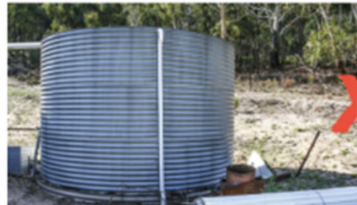
Sheltering in a water tank is NOT safe
